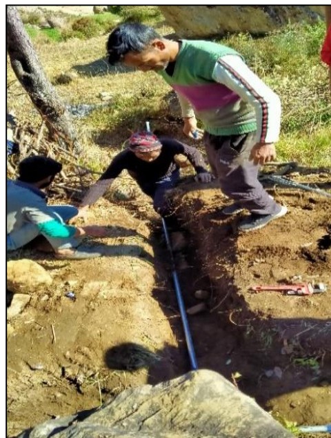
Layout of pipeline and installation of silting chamber
